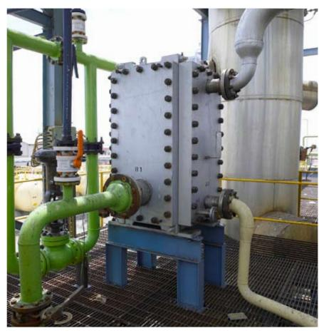
in its plants. The heat exchangers are used as condensers, reboilers, vaporizers and coolers.
