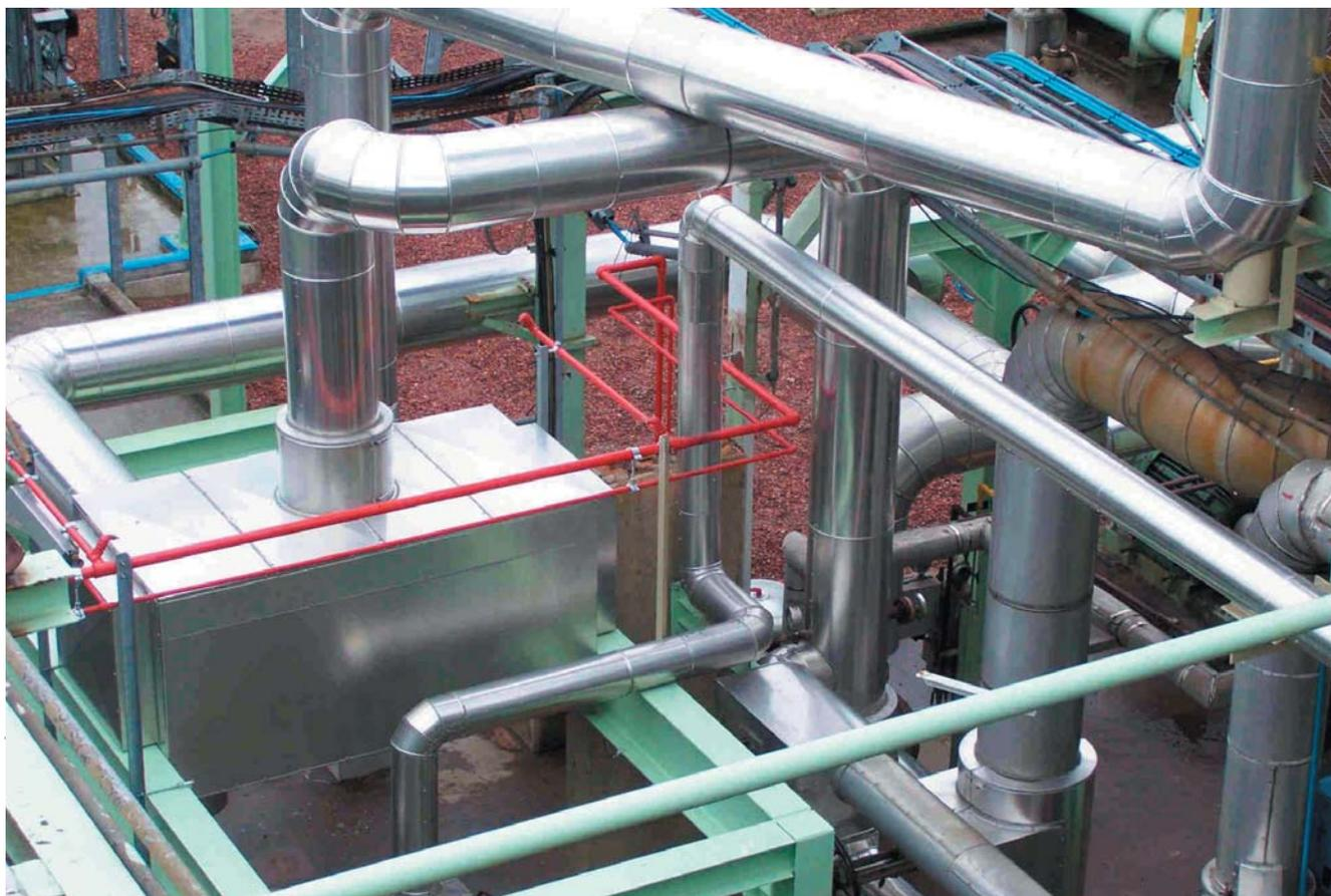
Operating as a reboiler in the solvent recovery column at Dow Wolff Cellulosics, Compabloc offers a substantial increase in capacity compared with the shell-and-tube heat exchanger it replaced.
