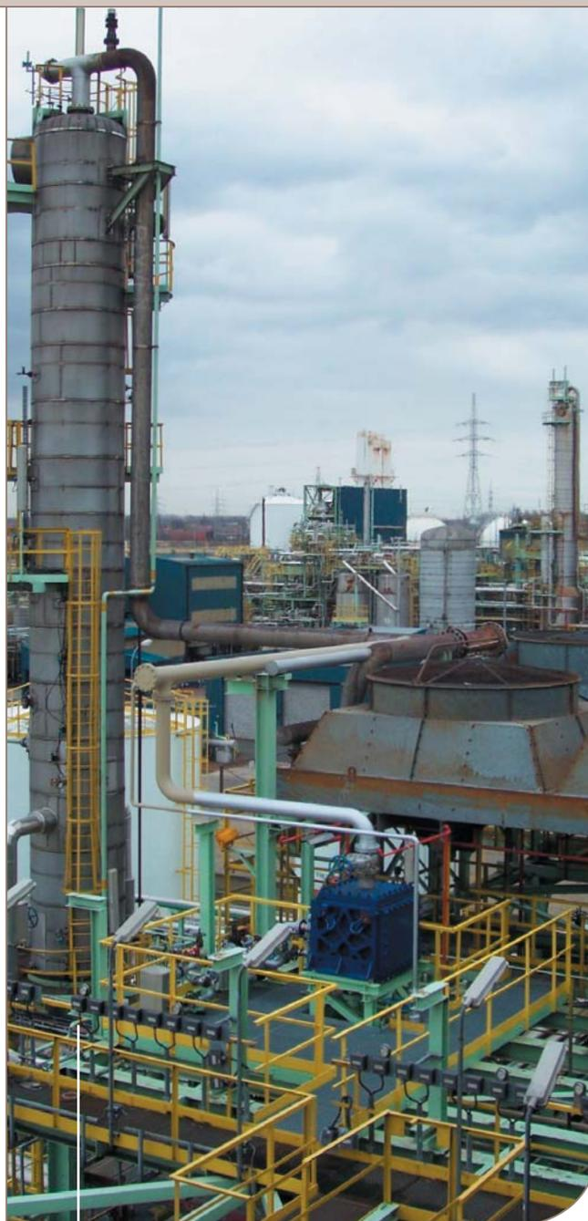
Installed as a condenser in a solvent recovery column at Dow Wolff Cellulosics, the Compabloc compact heat exchanger is visible next to the air coolers.
